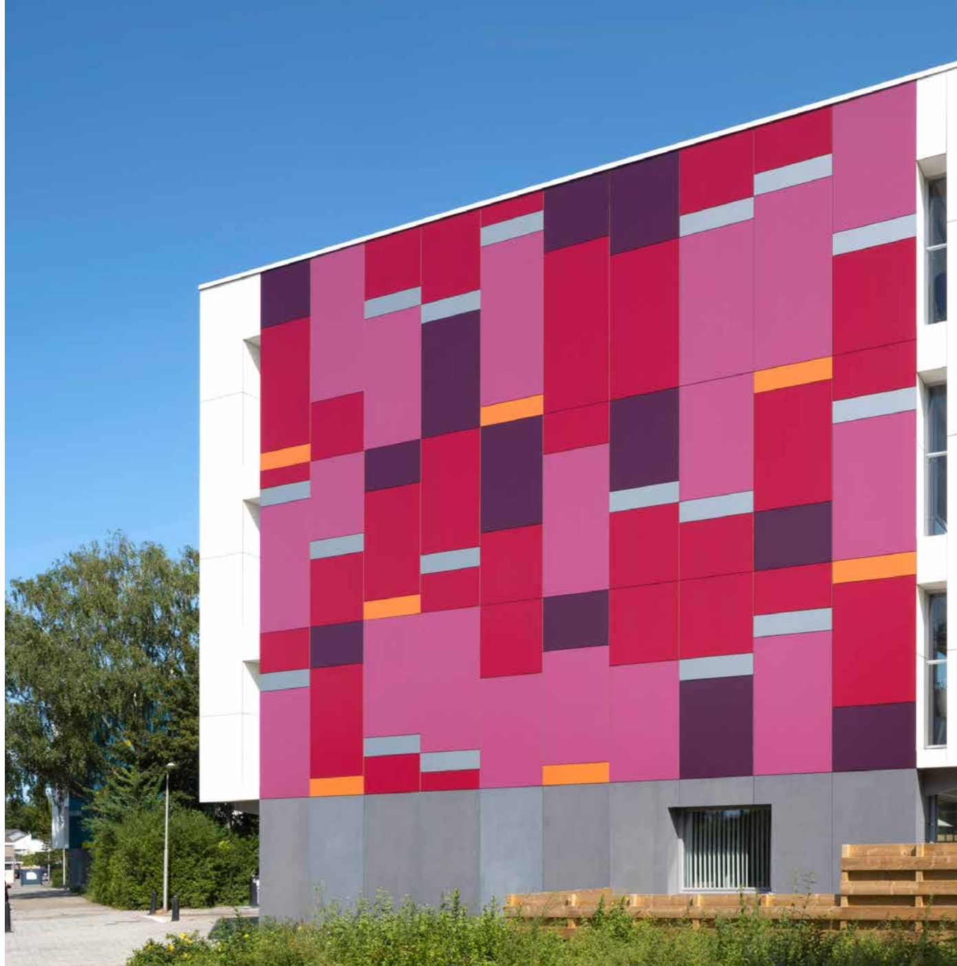
Project: Renovated flats, Emmeloord, The Netherlands
